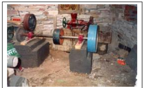
Foundation for counter shaft
