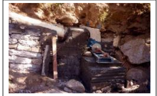
Generator & Turbine foundation
