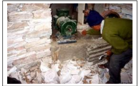
Installation of Generator
