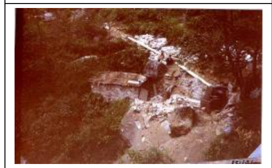
Installation of Penstock
