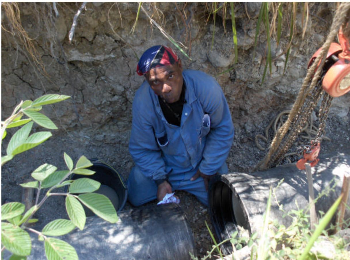
Figure 4.2 The Construction Manager preparing for jointing of ductile pipes Dia 400mm
